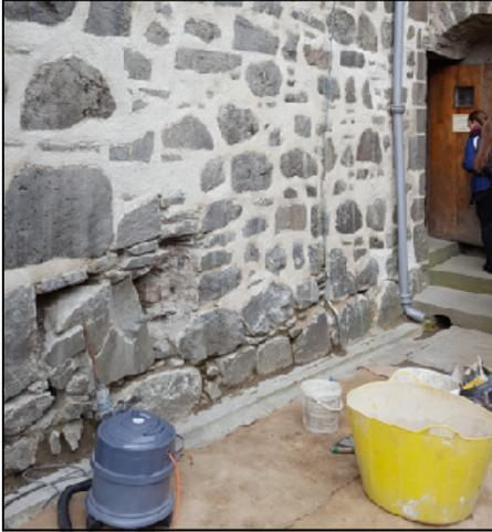
The voids (pictured left) that were opened up in the 5 meter thick Keep Wall were measured as up to 1 meter deep. All friable Easdale slate that had been used in between the large imperious stones had to be removed along with the hard cement mortar and replaced with Caithness stone and the new purpose made lime mortar.
